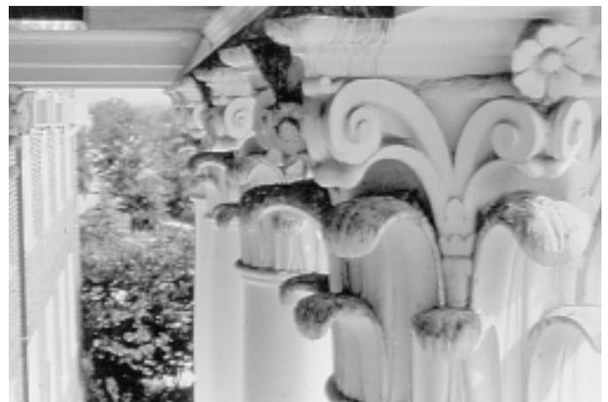
Figure 18.4. Defacement of building from pigeon droppings.
