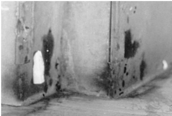
Figure 16.5. Rat droppings and grease marks.
