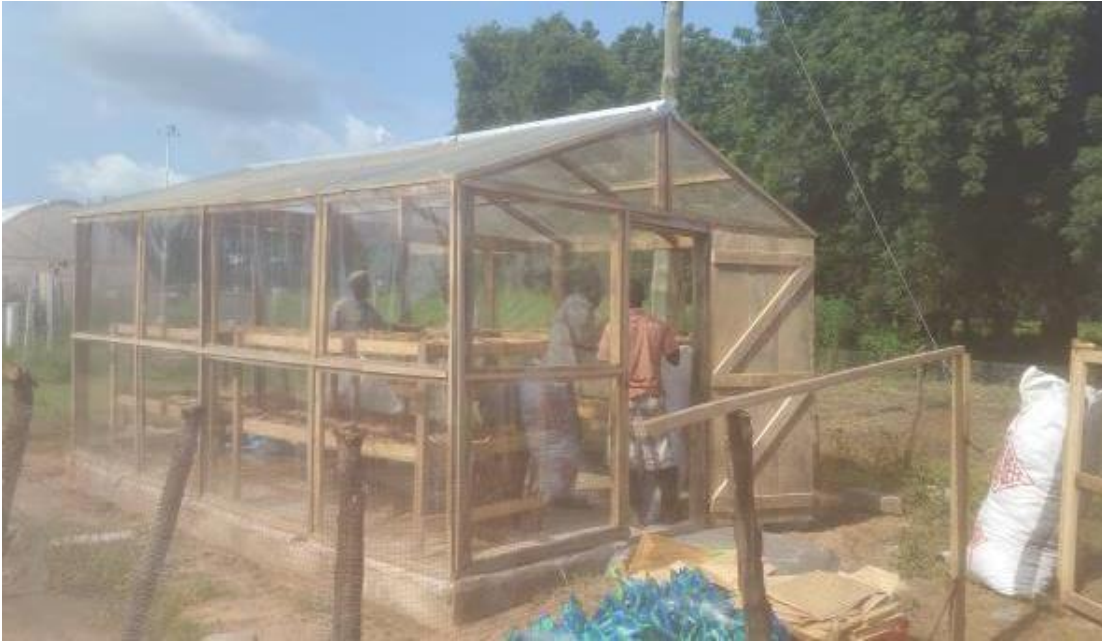
Figure 3. Greenhouse solar dryer using material from the LIL to facilitate drying of cowpea during the rainy season.
