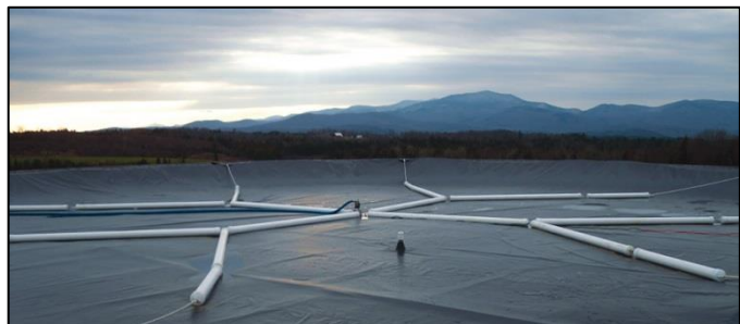
Figure 3. Biogas cover over digester vessel. Photo courtesy of UEM, Inc.
