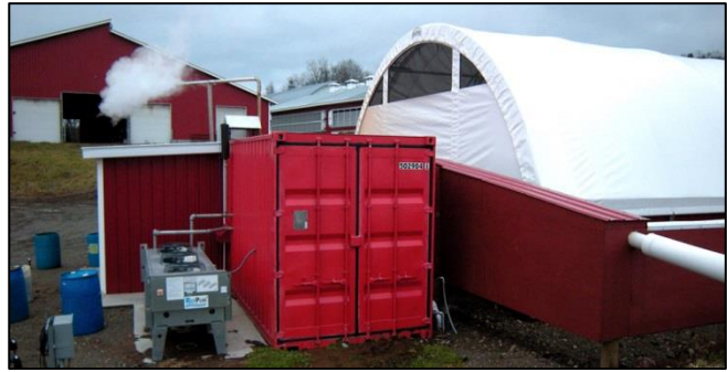
Figure 2. Storage container with solids separation equipment (foreground) and fiber storage shed (right). Photo courtesy of Nora Goldstein.
