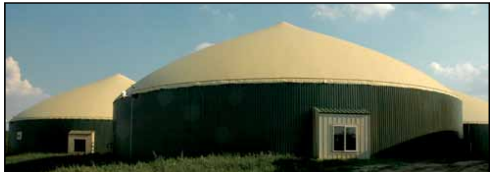
Green Meadow Farms, Inc., of Elsie, Mich. was the first newly constructed AD on a Michigan Farm in more than 20 years.
