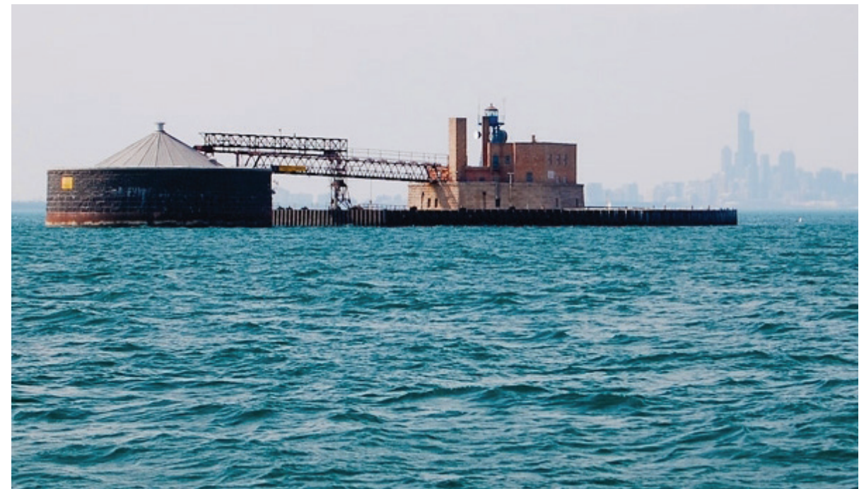
One of Chicago's water cribs, where water is pumped from Lake Michigan to supply parts of our region with drinking water. Photo Credit Eric Allix Rogers
