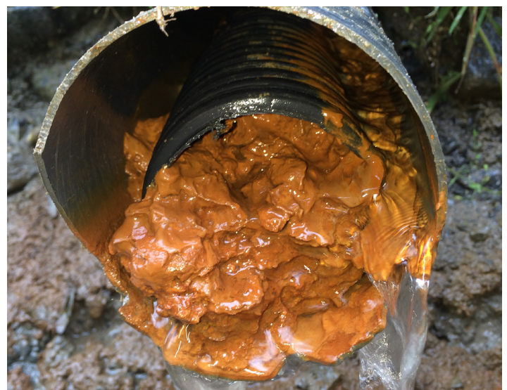
Figure 1- An extreme case of iron ochre deposits inside of a drain pipe (photo credit: Patrick Ruohy)
