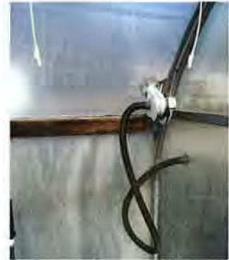
Providing outside air reduces moisture condensation between the plastic layers.
