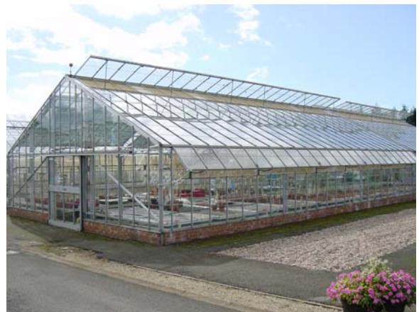
Figure 18. Natural ventilation in a glass-glazed greenhouse. Photo courtesy of A.J. Both, Rutgers University.
