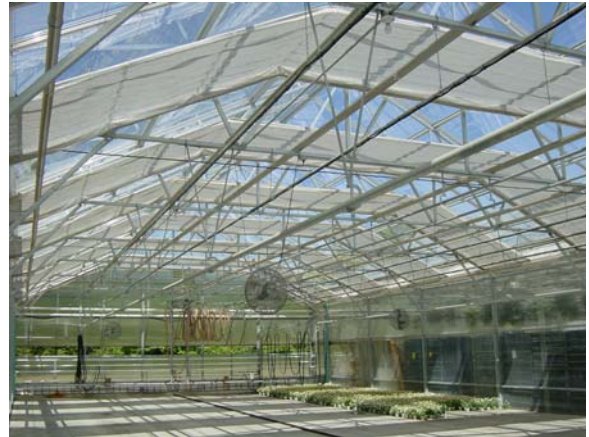
Figure 19. Example of an internal shade system in a greenhouse. Photo courtesy of A.J. Both, Rutgers University.
