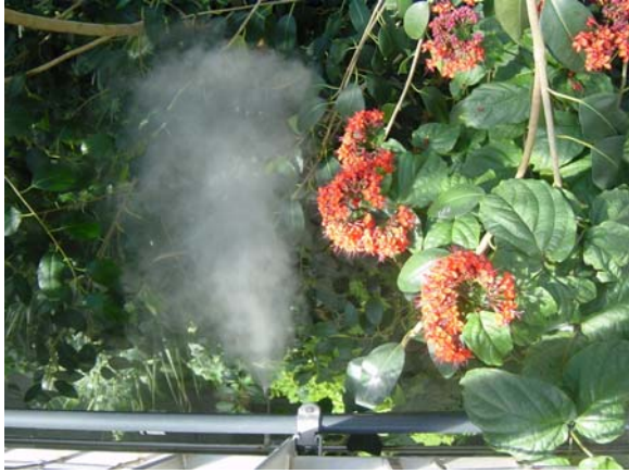
Figure 21. Top-down view of a fog nozzle delivering a small-droplet mist for evaporative cooling. Photo courtesy of A.J. Both, Rutgers University.
