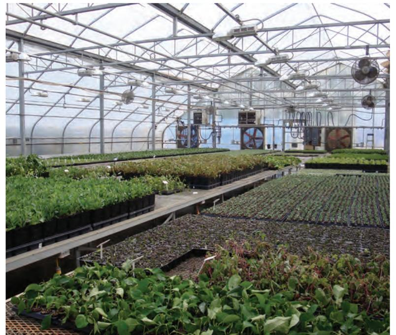
Figure 1. HPS fixtures and HAF fans are examples of acronyms commonly used in CEA.
