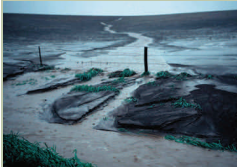
Sediment loading into drainage ditch
