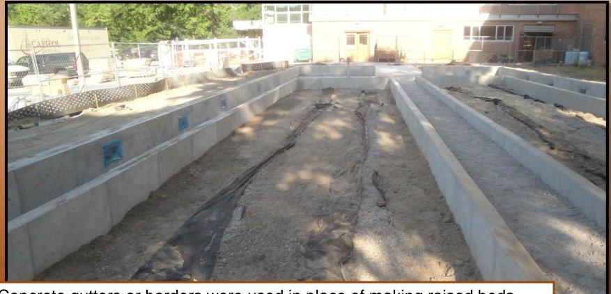
Concrete gutters or borders were used in place of making raised beds with wood borders. The permanent borders may also provide heat retention. Fabric in this picture is covering drain tile placed in gravel. The beds were lined with landscape fabric prior to installing the compost. The walkways are crushed gravel for solid footing and drainage.
