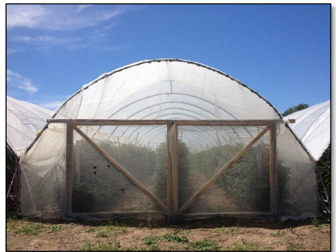
Fig. 4 Exclusion netting fitted to a high tunnel raspberry system, with doors to allow for sprayer access.
