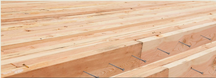
Nail-laminated timber (NLT)
