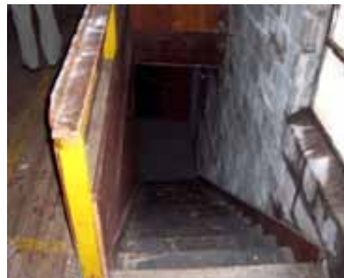
Figure III-25: Staircase leading to Second Floor 21035 Van Dyke Avenue
