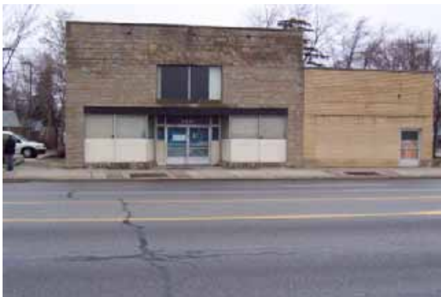
Figure III-23: Peacock Building from Van Dyke Avenue
