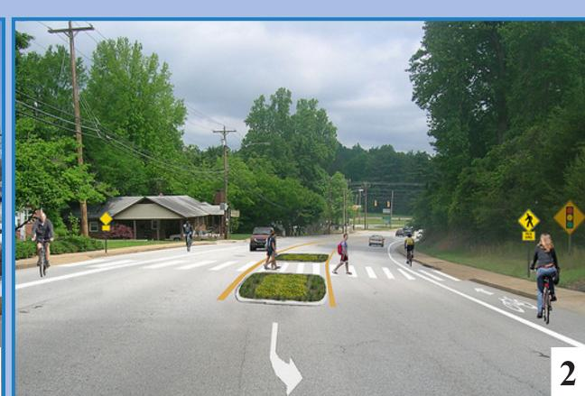
Image 1 shows a block of southbound Gratiot that does not provide pedestrians with a midblock crosswalk. Midblock crosswalks reduce the distance a pedestrian has to travel to reach a safe or signalized crosswalk. The image also shows that there are inadequate facilities to accomodate non-motorized transportation options. Image 2 provides an example of a midblock crosswalk option with non-motorized transportation options in Easley, SC.
