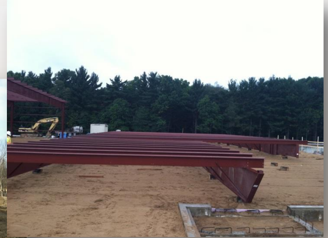
Prefabricated Soffit Sections and Roof Bays- Four Winds Casino
