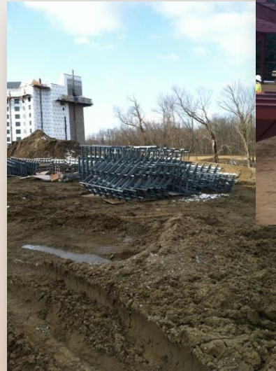
Prefabricated Soffit Sections and Roof Bays- Four Winds Casino
