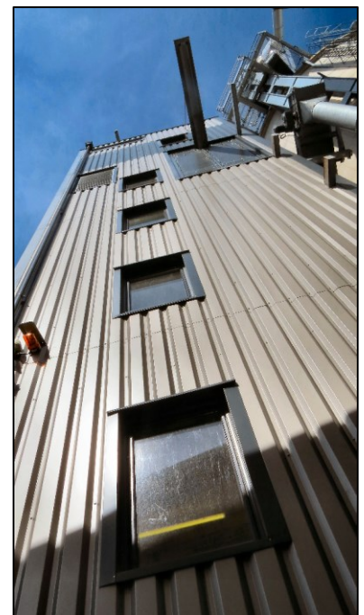
Vertically-oriented, gravity-engaged pellet plant, with hammermill and pellet press.
