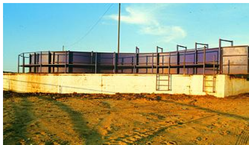
Level dock loading/offloading facility
