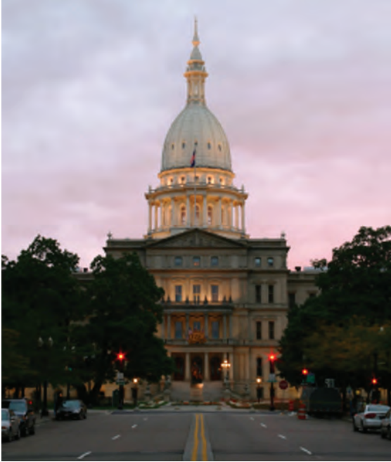
The Michigan State Capitol building in Lansing.
