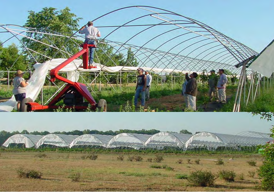
Figure 1. Haygrove tunnels at the Southwest Michigan Research and Extension Center; under construction (top) and complete (bottom).
