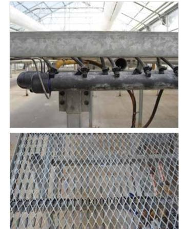
Figure 1. Root-zone heating of benches can be useful during propagation. A common temperature target for the media is 73 to 77° F. (Photos: Roberto Lopez, Purdue University)
