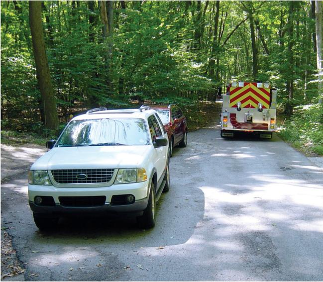
**Figure 3.** Passing areas on narrow lakeshore private roadways such as this one near Grand Haven, Mich., allow emergency vehicles to pass. (Courtesy of Grand Haven Township Fire and Rescue)
