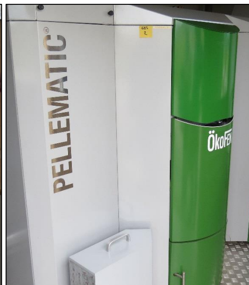
Home-styled pellet storage bin and fully automatic pellet boiler.
