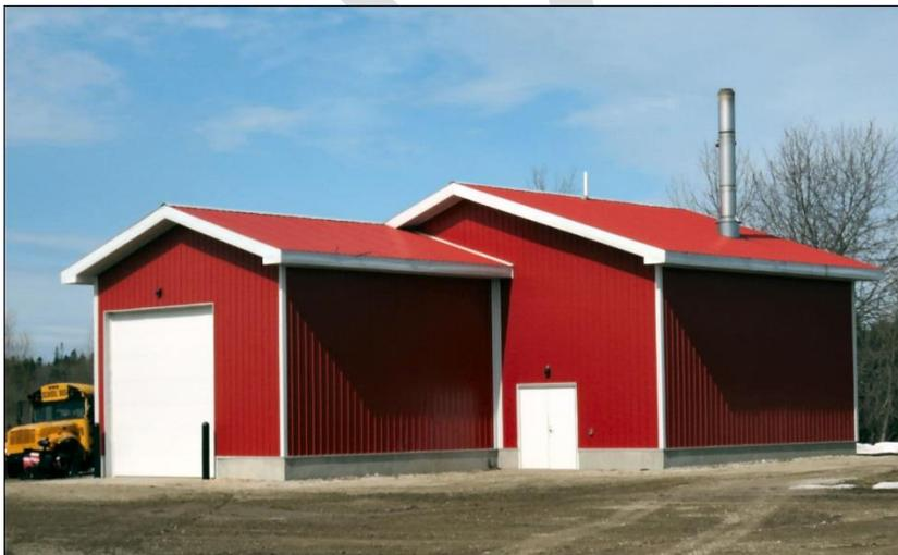
A new building was constructed to house the new heating system and to hold chips. Chip trucks and vans back into the storage area for unloading. A walking auger moves chips from the storage area floor into a conveyor trough. The conveyor moves wood chips into the boiler metering bin where fuel is added to the boiler as computer controls dictate.
