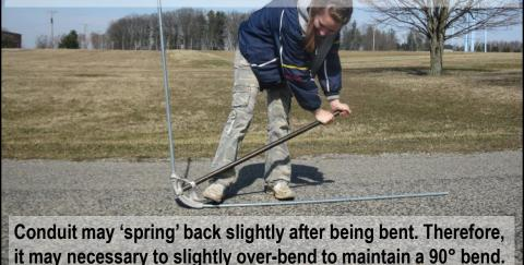
The first and third marks (each 2 ft from opposite ends of the pipe) made at the beginning of the process are visible at the top-center and right-center of the image. Each locate where a 45° bend will be made to form the sidewall.
