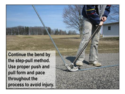
Complete the bend by stopping at the correct angle (in this case, 90°). The bar of the bender should be only slightly above the line that bisects the peak of the frame.
