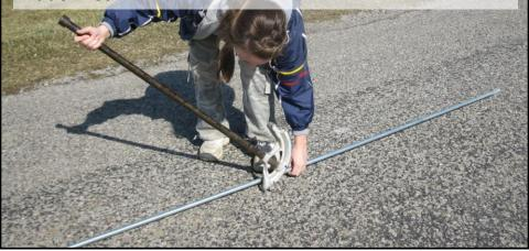
Align the correct positions on the bender and pipe. On this conduit bender, the 5 ft (90° peak bend) mark is aligned with the arrow.
