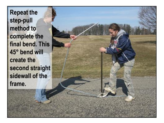
Complete the bend by stopping at the correct angle. The bar of the bender should be only slightly above the line that bisects the turn from the frame's sidewall to its roof.
