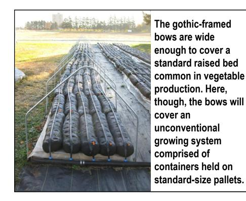
Bows are in place and covering has begun. Here, 12-ft wide x 80 ft long sections of 6-mil greenhouse film are secured with cement blocks. Additional steps are required to secure the plastic where high wind and heavy snow is expected.
