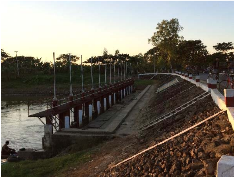
Water control infrastructure, Maubin township
