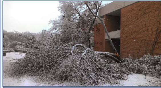
Ice storm damage, Winter 2013
