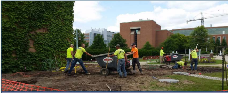
Construction begins, July 2015
