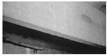
Figure 6.2. Anobiid beetle damage in pine floor joist—note frass being pushed out of old exit holes (USDA Forest Service).
