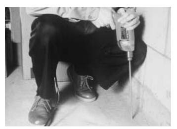
Figure 3.5. Slabs are drilled so that termiticide can be injected through holes to treat the soil beneath.
