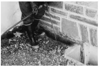
Figure 4.7. A typical basement treatment will also include trenching and rodding the outside perimeter of the foundation.
