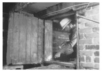
Figure 3.9. Inspection of crawl space for termite infestations (he should also be wearing gloves).
