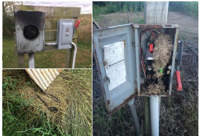
**Figure 10.** Mice, snakes, and other small vermin squeeze into electric boxes for shelter.
