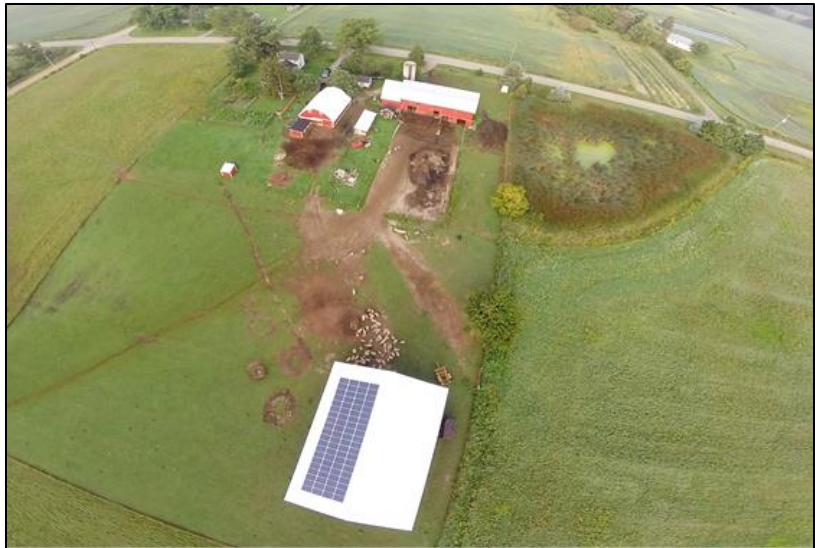
Figure 2. Solar panels on barn. Credit: Kinder Engineering.
