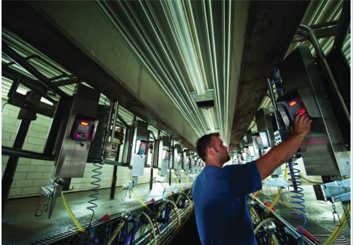
State-of-the-art robotic milking parlors like this one have helped reduce the occurrence of mastitis in Michigan. These modern-day facilities are well-ventilated and help to keep the cows clean, dry and comfortable.
