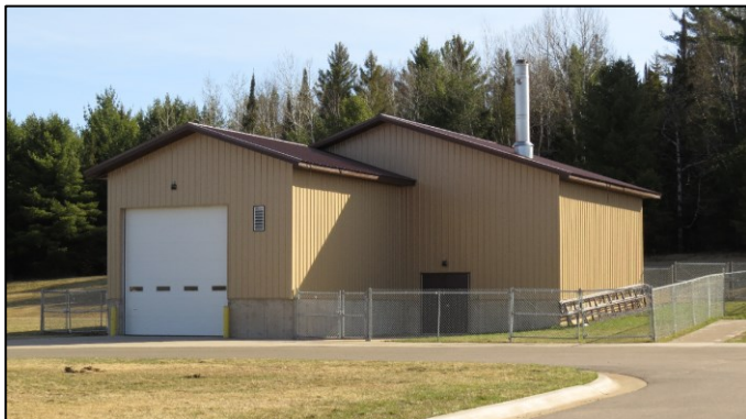
Heating plant and chip storage building.
